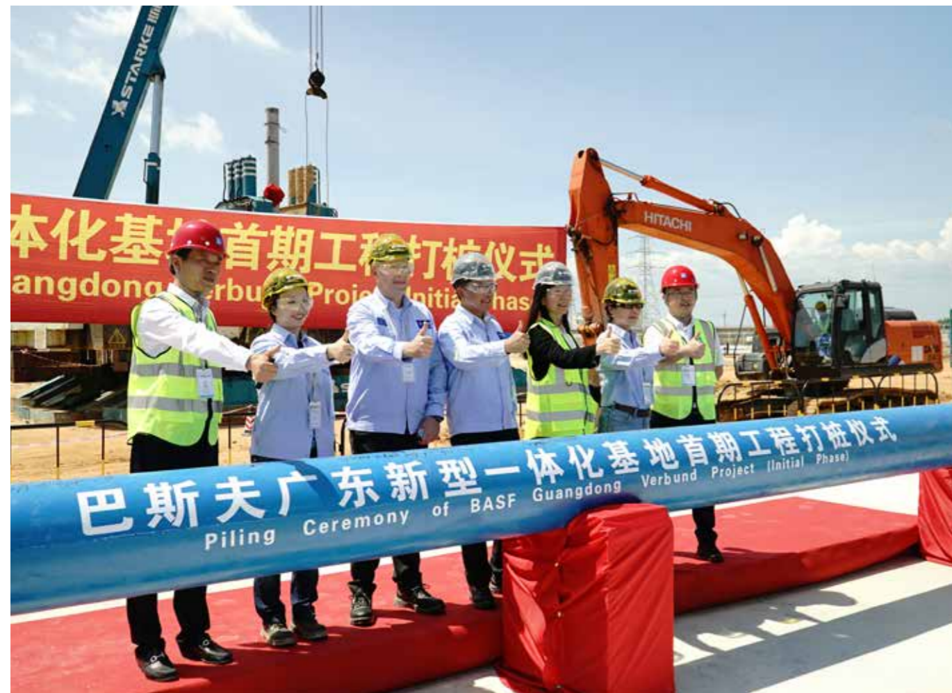
BASF started piling for the first plants of its Zhanjiang Verbund site.
