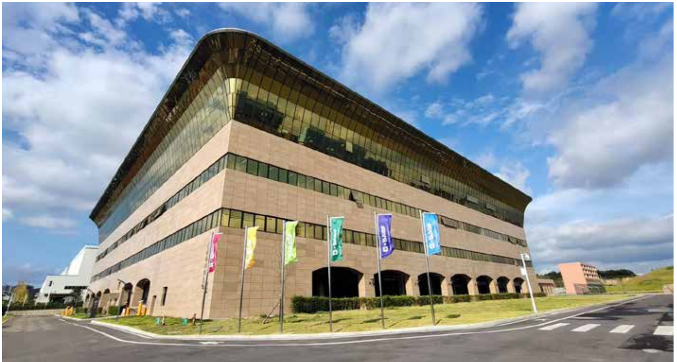
BASF Shanshan Battery Materials has built up the advanced R&D center at Da Changsha Site in Hunan.
