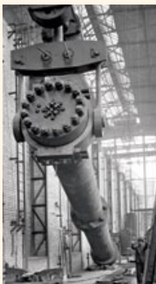
A high-pressure reactor being built into the ammonia plant in 1921.
