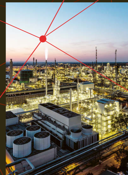
In a joint effort with SABIC and Linde, BASF is constructing the world's first demonstration plant for electrically heated steam cracker furnaces at its Ludwigshafen site in Germany.
