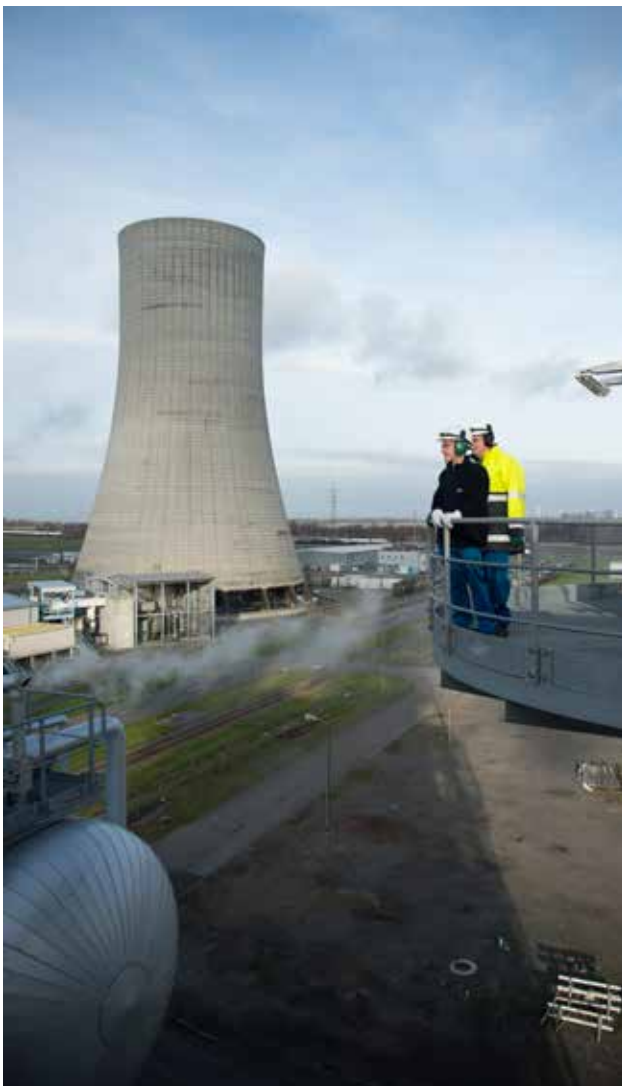
Two employees have a good overview of Zandvliet Power's cooling tower.
