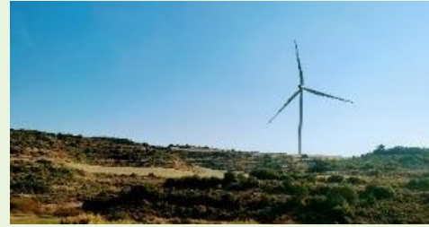
25 years onshore wind power from Spain
