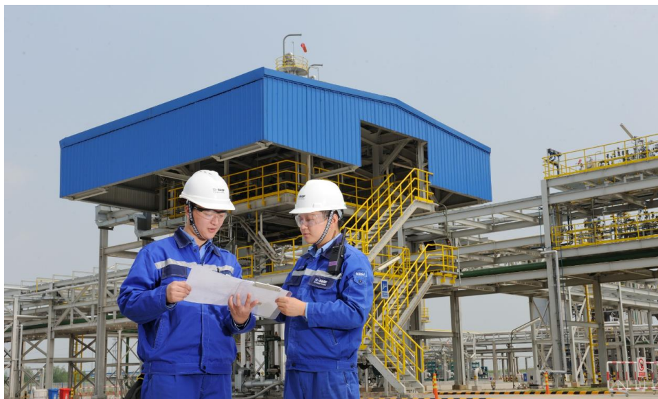
BASF PEA/ DMAPA amines plant in Nanjing, China
