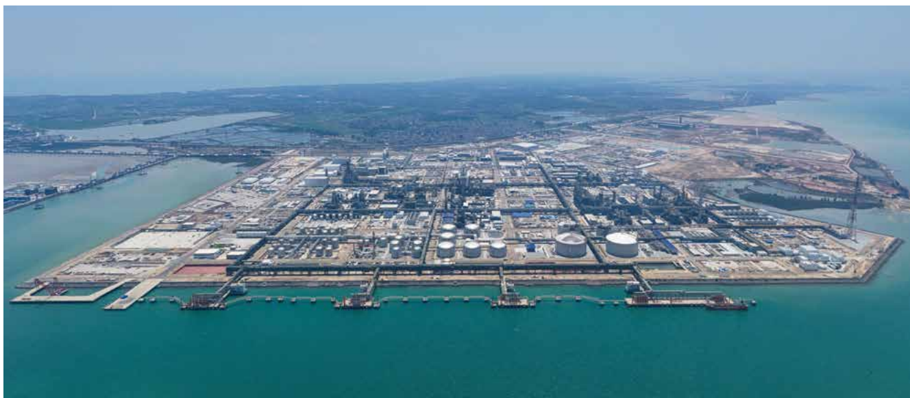
Construction in progress at BASF's Zhanjiang Verbund site (status April 2025)
