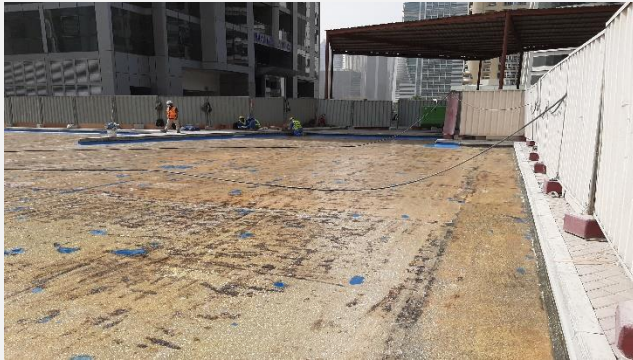
Before -Elastocoat application
