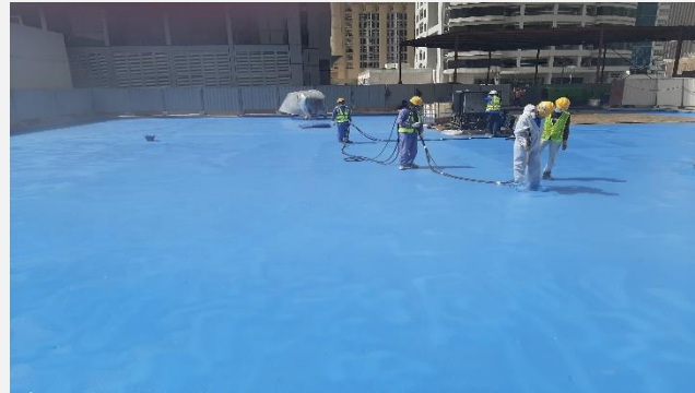
After – Elastocoat application
