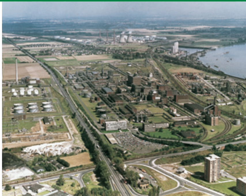
Entering the age of oil together: BASF builds ROW, a plastics production facility, in collaboration with Shell in Wesseling.
