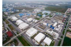
BASF inaugurated automotive coatings plant in Shanghai
