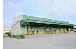
BASF opened its first automotive coatings plant in Thailand
