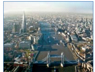
Europe's second tallest building: after completion, the Shard in London will have a height of 310 meters. Photo: Sellar Property Group
