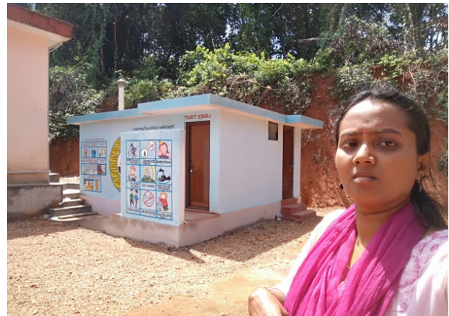
Girls' toilet at Mangalore School
