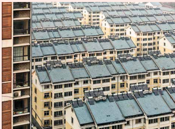
China harnesses the power of the sun: The Sun-Moon Mansion in Dezhou is the world's largest solar-operated building (top picture). Collectors are inexpensive and in the cities many residents use warm water that has been heated by the sun (bottom picture).
