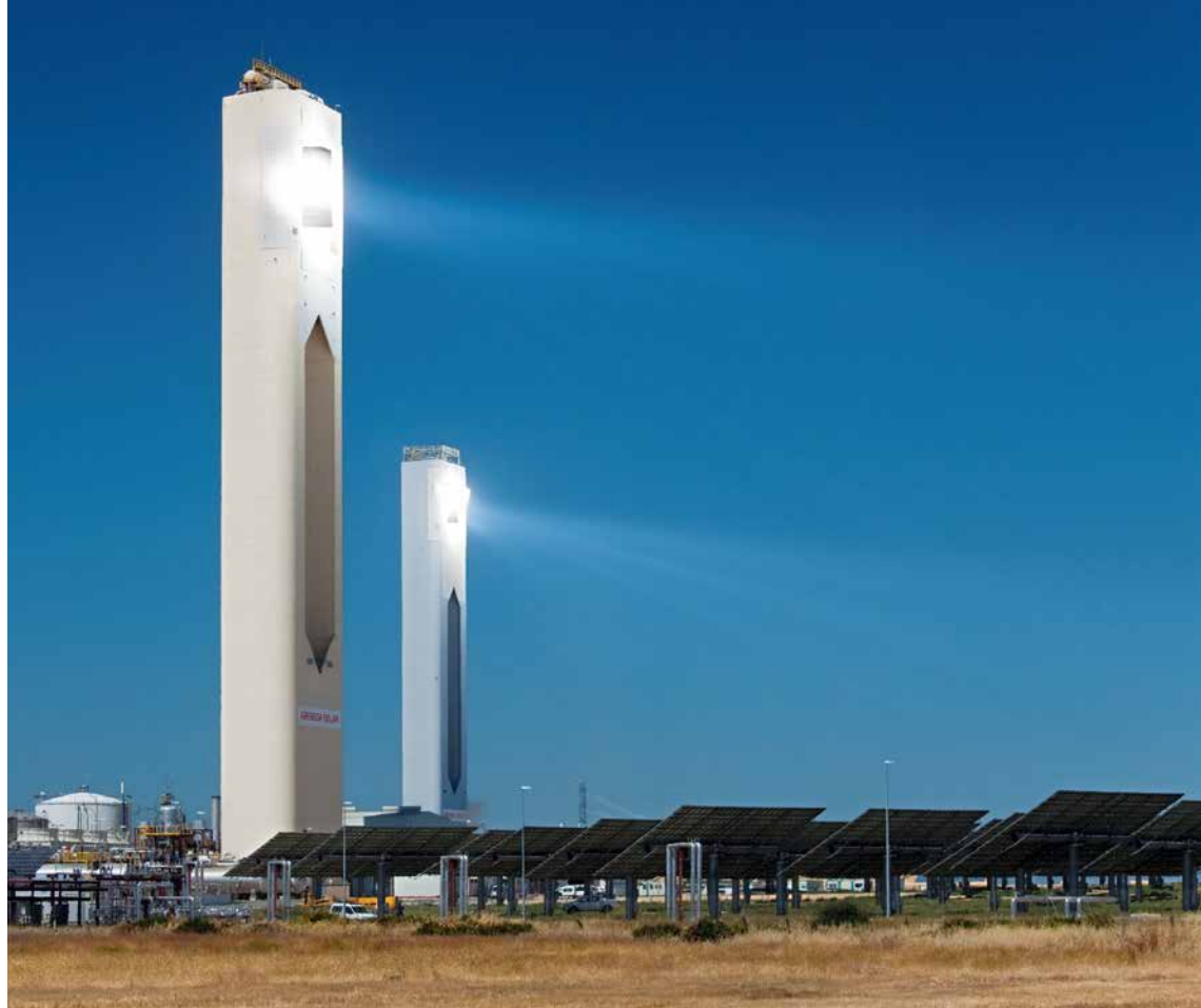
Solar towers achieve the highest thermal efficiency. The PS20 power plant belonging to the company Abengoa Solar in Seville, Spain, has an output of 20 megawatts.
