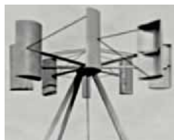
Above In 1887, Scotsman Professor James Blyth built the first ever wind turbine for power generation. Eight years later came a second, improved design, which provided emergency power for 30 years to the psychiatric clinic in Montrose/Scotland.
